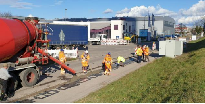
Electreon laying a wireless road in Germany. Electreon
