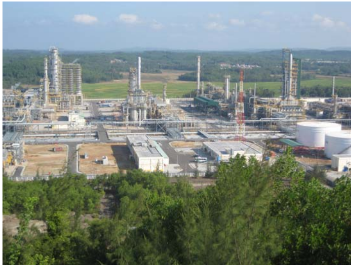
Dung Quat refinery
